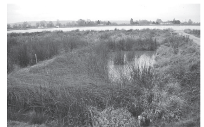
A pilot-scale constructed wetland at the city of Stanwood’s wastewater treatment facility, Snohomish County. Shown are two Scirpus acutus (bulrush) dominated marsh components, separated by a gravel berm.
